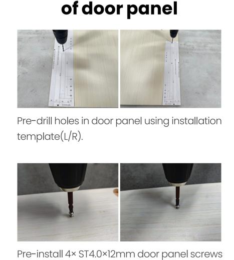
(do not fully tighten - leave 5mm gap for
